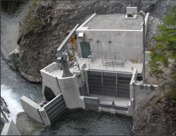
Cordova: Humpback Creek Hydro
